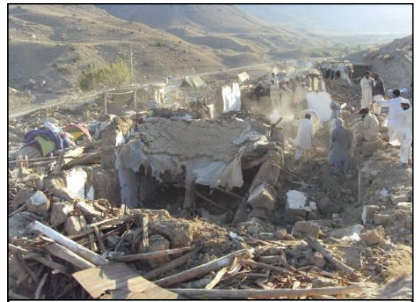
Wall and roof collapse at Kili Wam, Pakistan, October 2008. Courtesy of UN-Habitat, Pakistan
